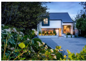
Passive House at Wayside Cork, Ireland
